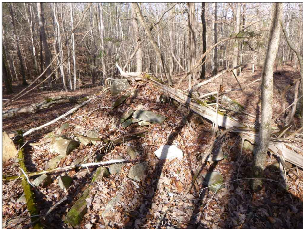
Figure 5.22. View of collapsed fieldstone chimney at site 38FA667, facing west.
