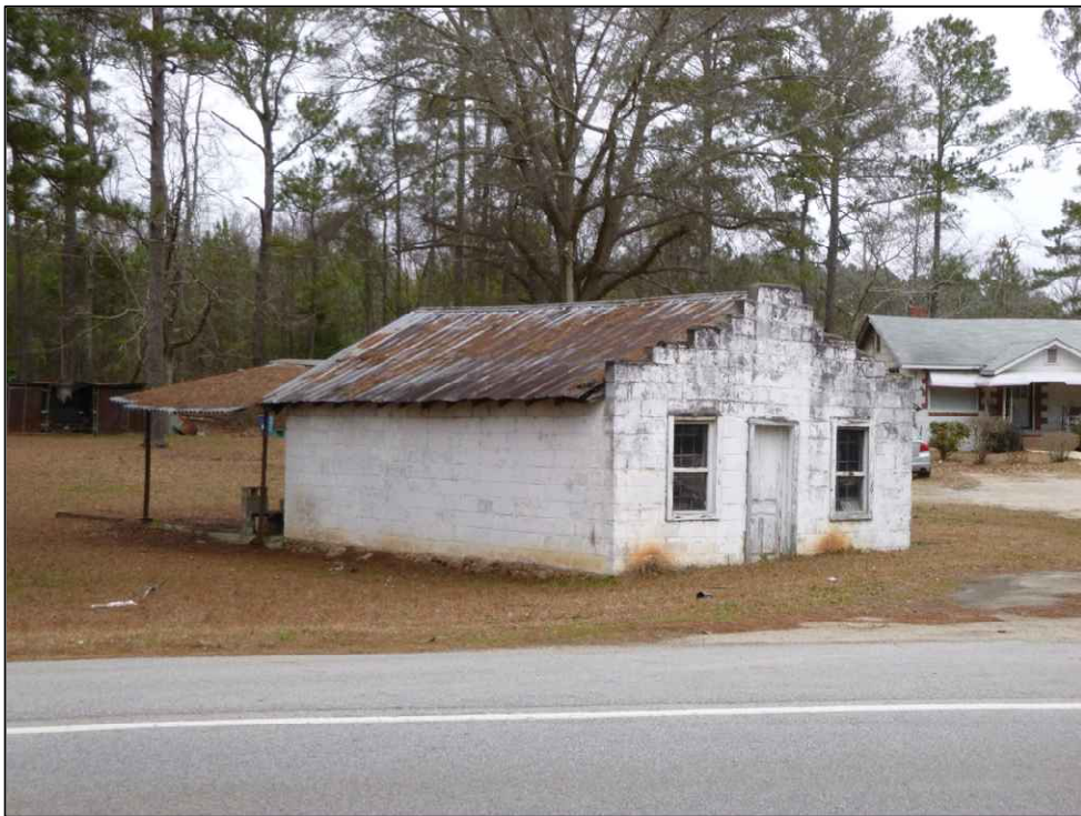
Figure 5.38. SHPO Survey Number 0109.1, facing north.
