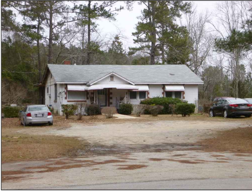
Figure 5.36. SHPO Survey Number 0109, facing north.
