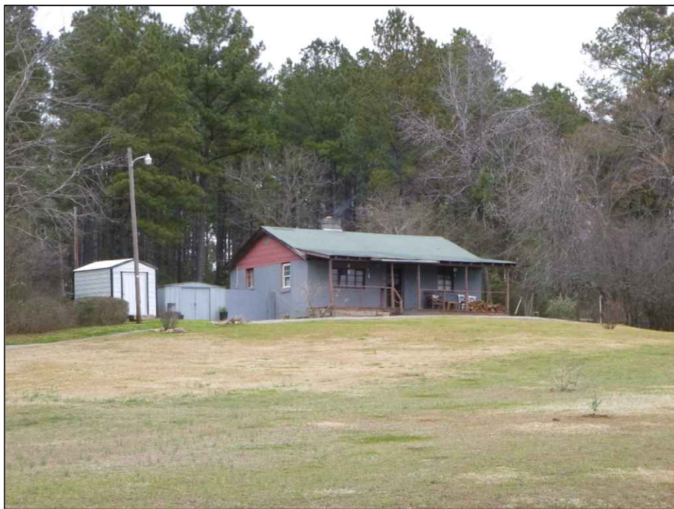
Figure 5.35. SHPO Survey Number 0108, facing north.
