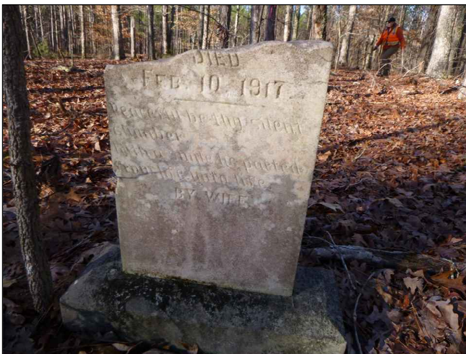
Figure 5.56. Damaged stone marker of Haywood F. Broom in the Old Homer Baptist Church Cemetery (SHPO Survey Number 0113; Site 38FA670), facing east.
