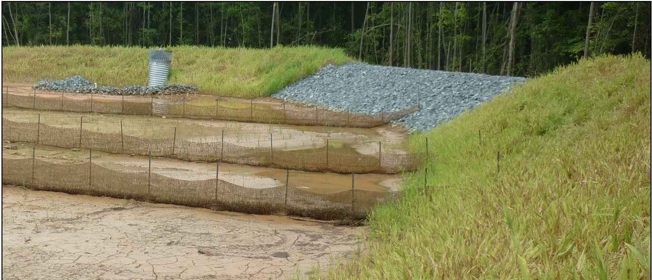
Photo: Porous Baffles
