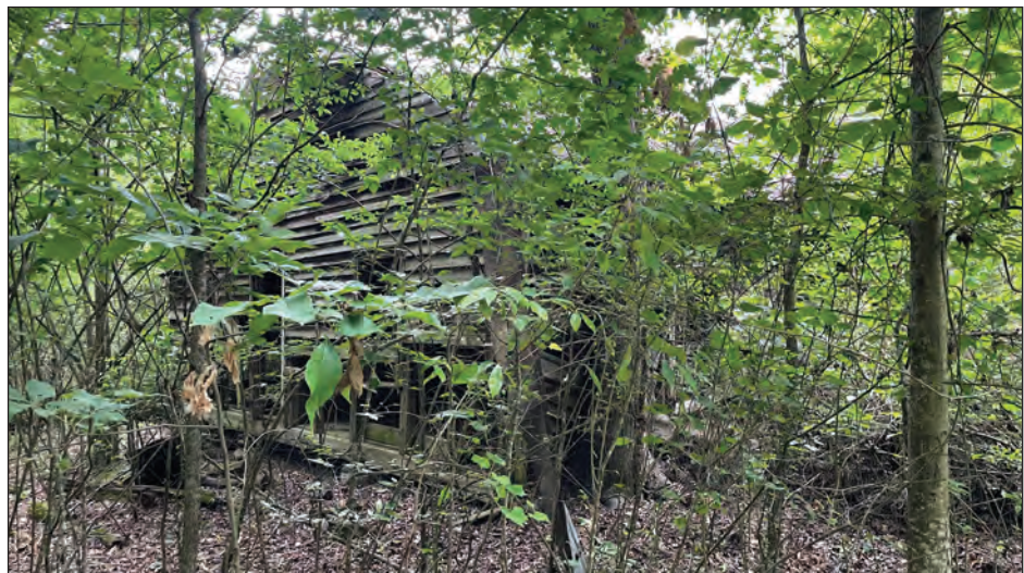
B. Frame House, Southeast, Facing Southeast
