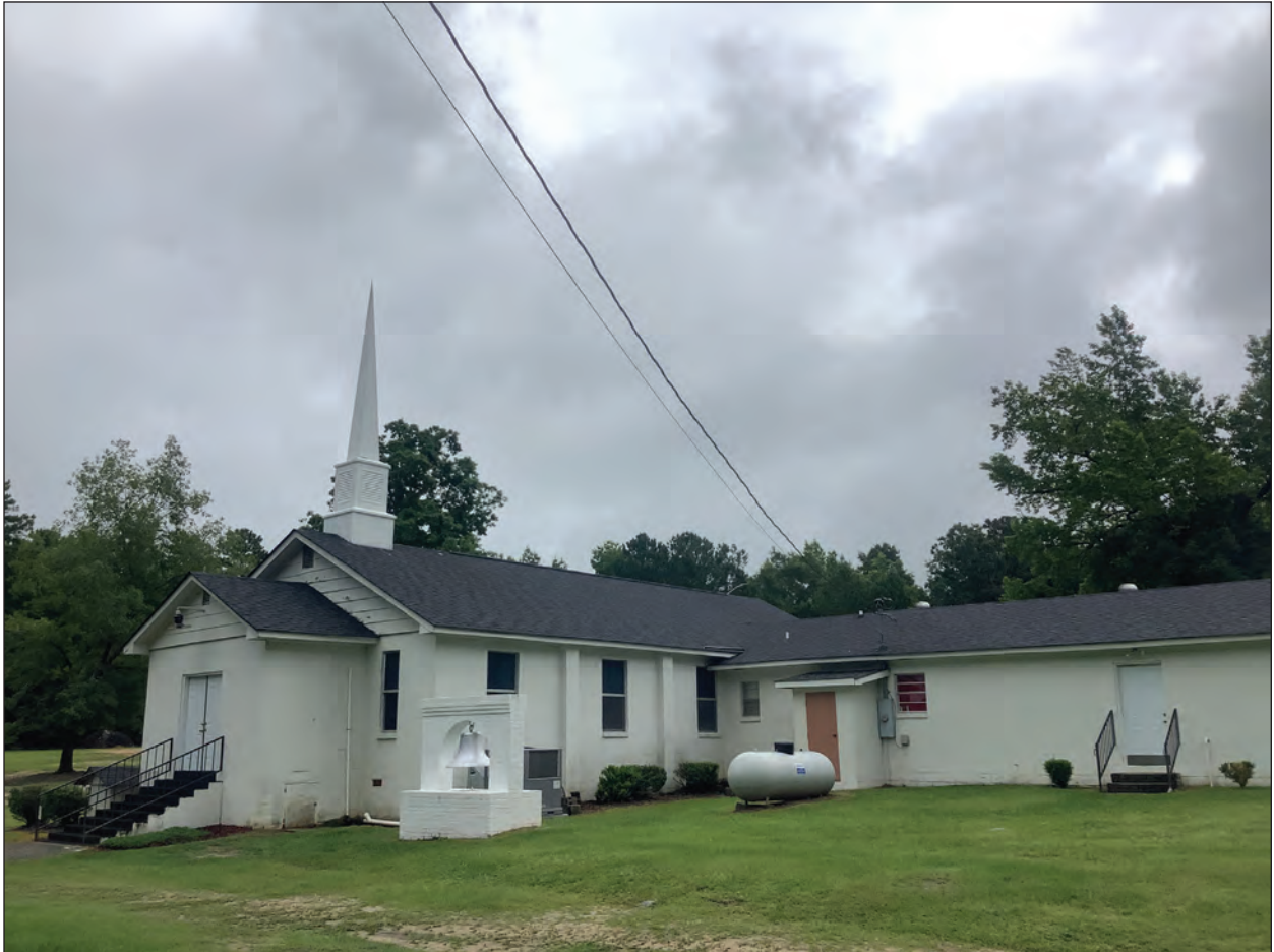
Figure 33. Resource 0053: Historic Core and South Wing of Church, Facing Northeast
