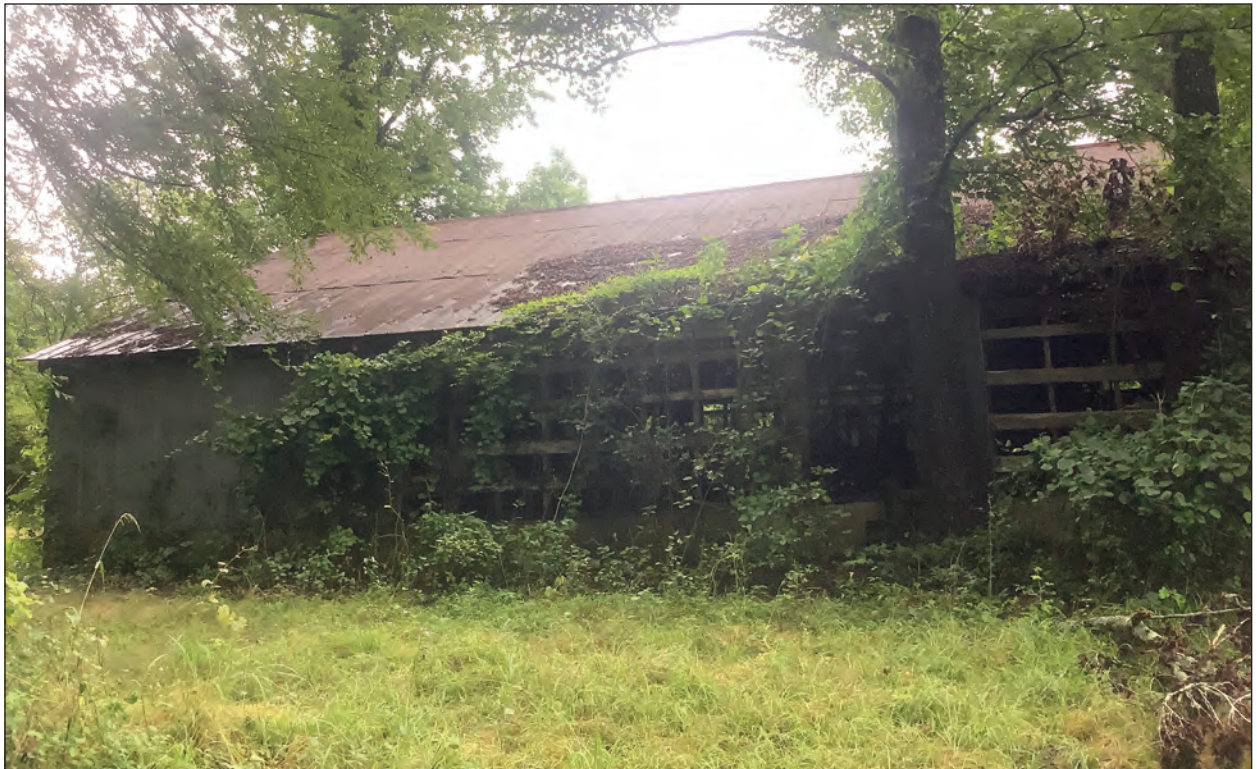
B. Southeast Elevation of Barn, Facing Northwest
