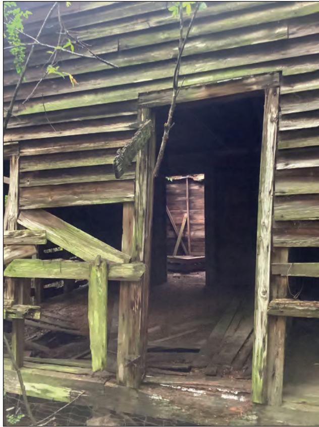
Figure 36. Resource 0055: Residence, West of Double Bridges Road
