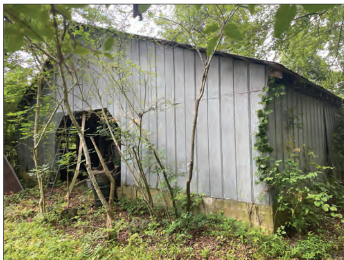
C. Barn, Facing Northeast
