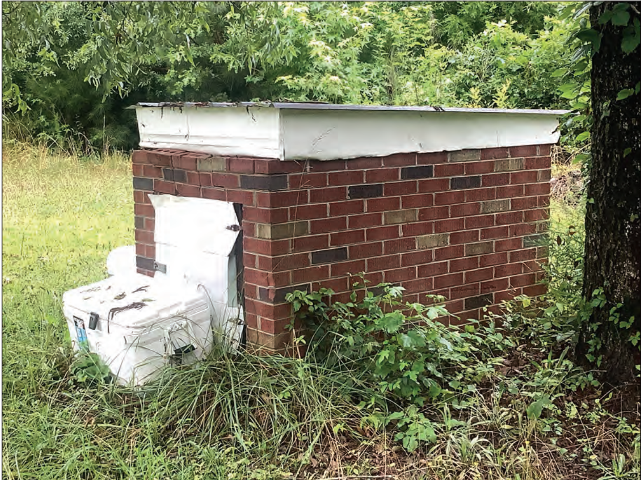
Figure 41. Resource 0056.01 Well/Pump House
