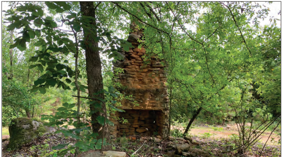
B. Chimney 2, Facing North
