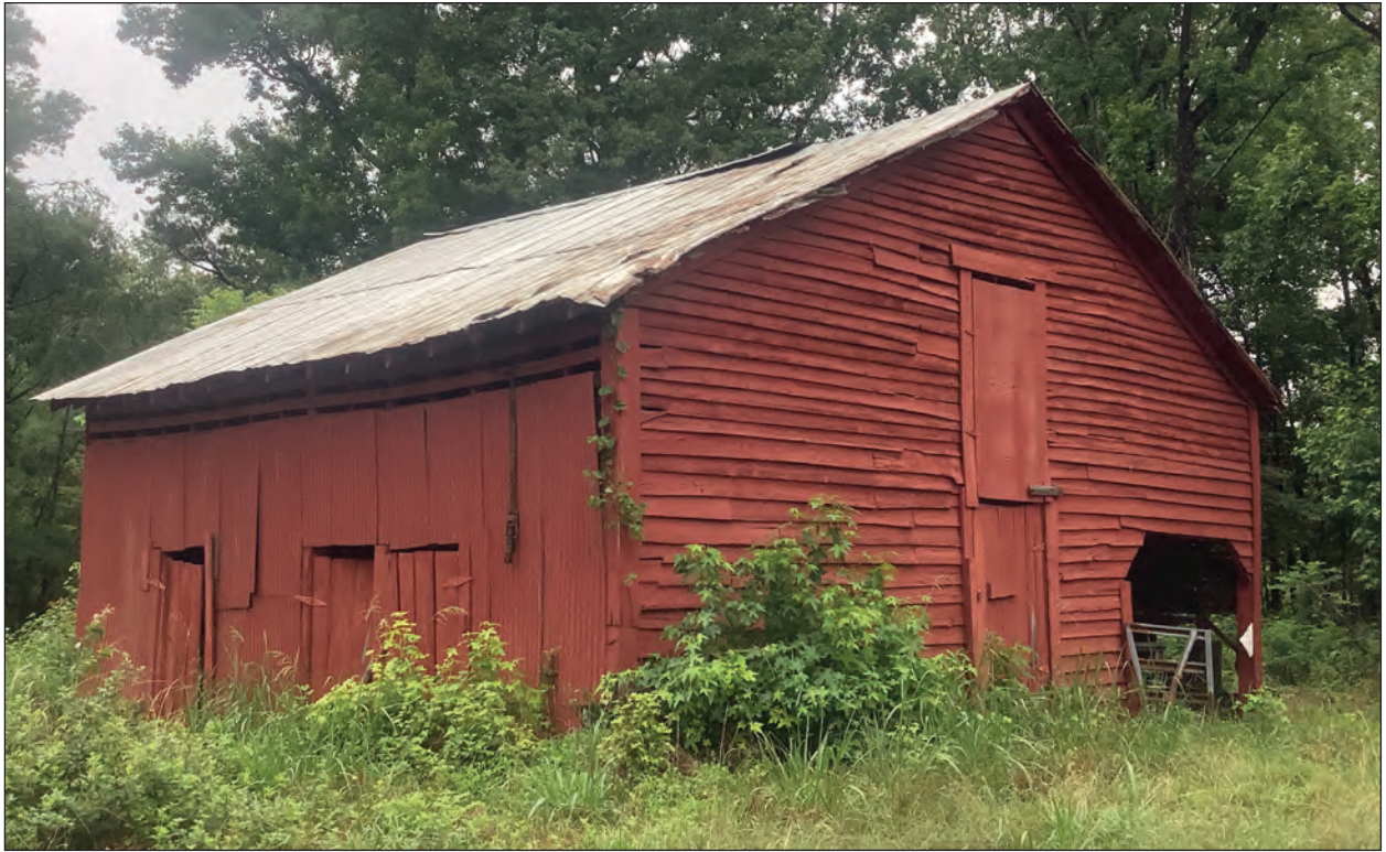
A. Northwest Oblique of Barn, Facing Southwest
