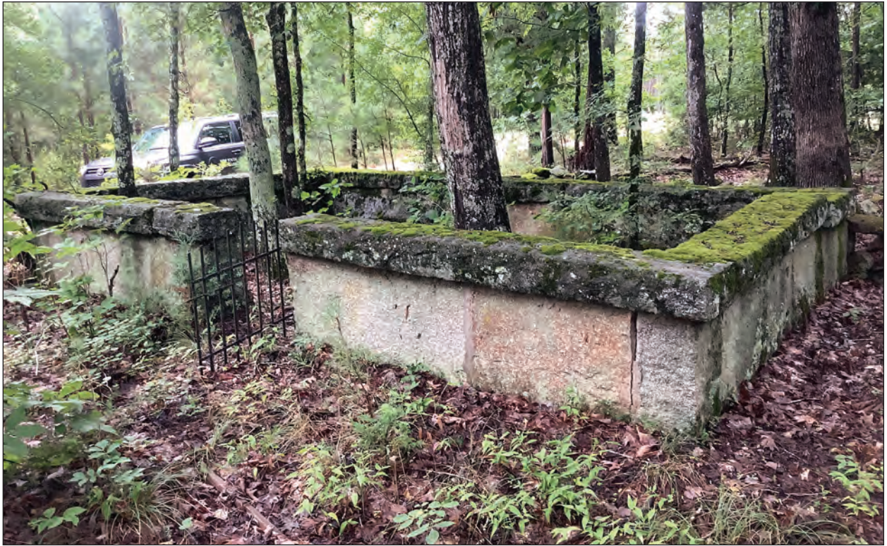
A. Main Enclosure, Facing Northeast
