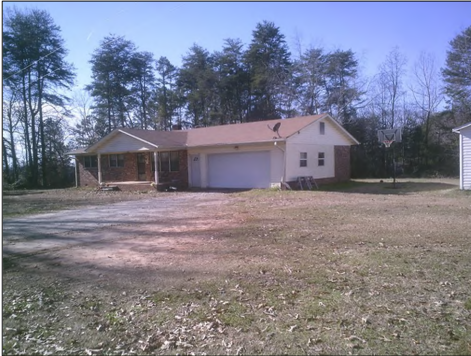
Figure 5.63. SHPO Site Number 1721 facing southwest.
