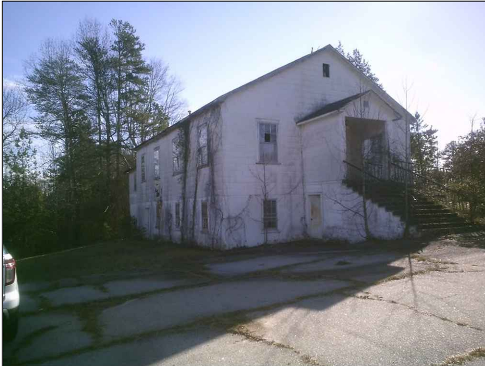
Figure 5.68. Hammett Grove Baptist Church (SHPO Site Number 1723), facing southeast.
