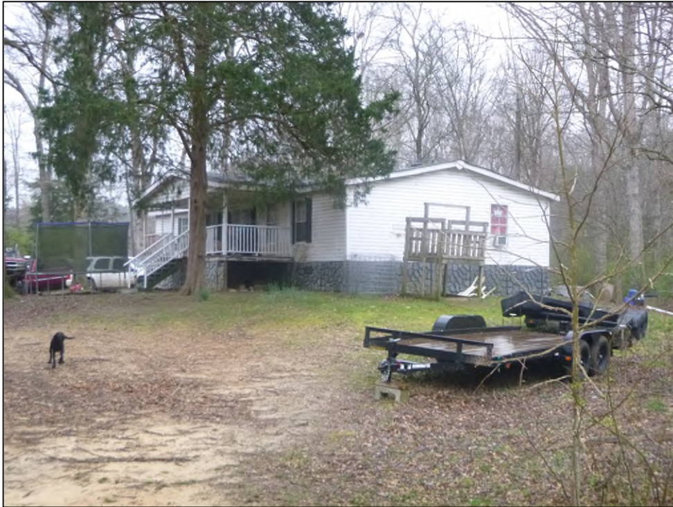
Figure 2.7. Typical structure within the project area, facing southwest.
