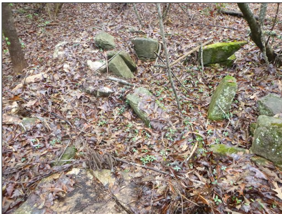
Figure 5.47. Lee Cemetery (38SP485/SHPO Site Number 1716), collapsed crypt, facing east.
