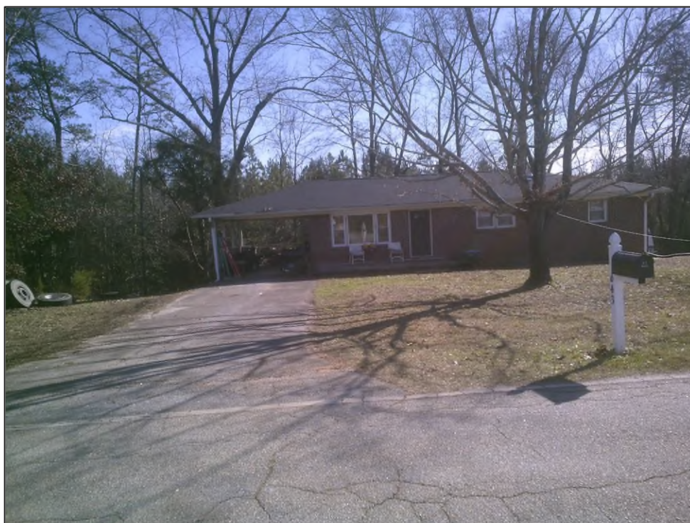
Figure 5.80. SHPO Site Number 1726, facing east.
