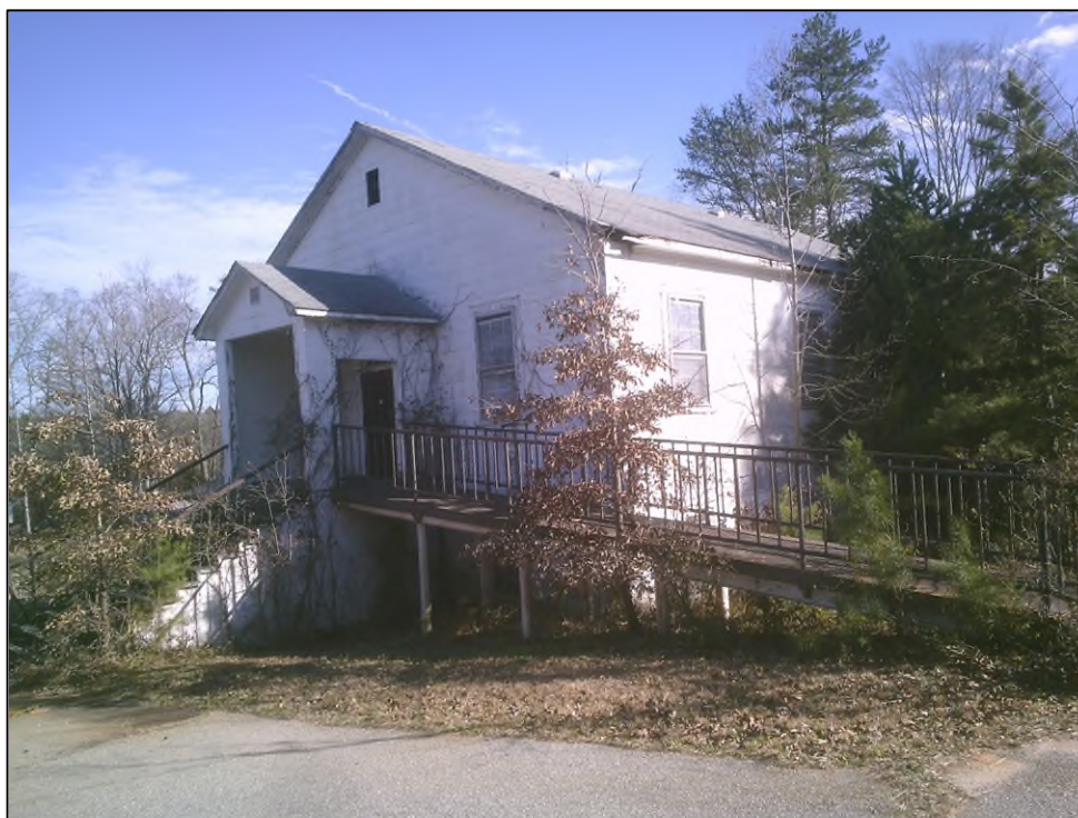
Figure 5.70. Hammett Grove Baptist Church (SHPO Site Number 1723), facing northeast.
