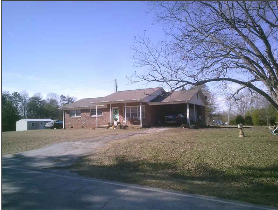
Figure 5.85. SHPO Site Number 1727, facing southwest.
