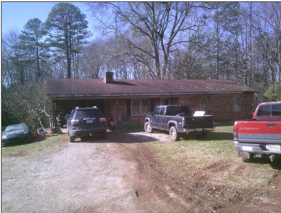
Figure 5.55. SHPO Site Number 1718, facing south.
