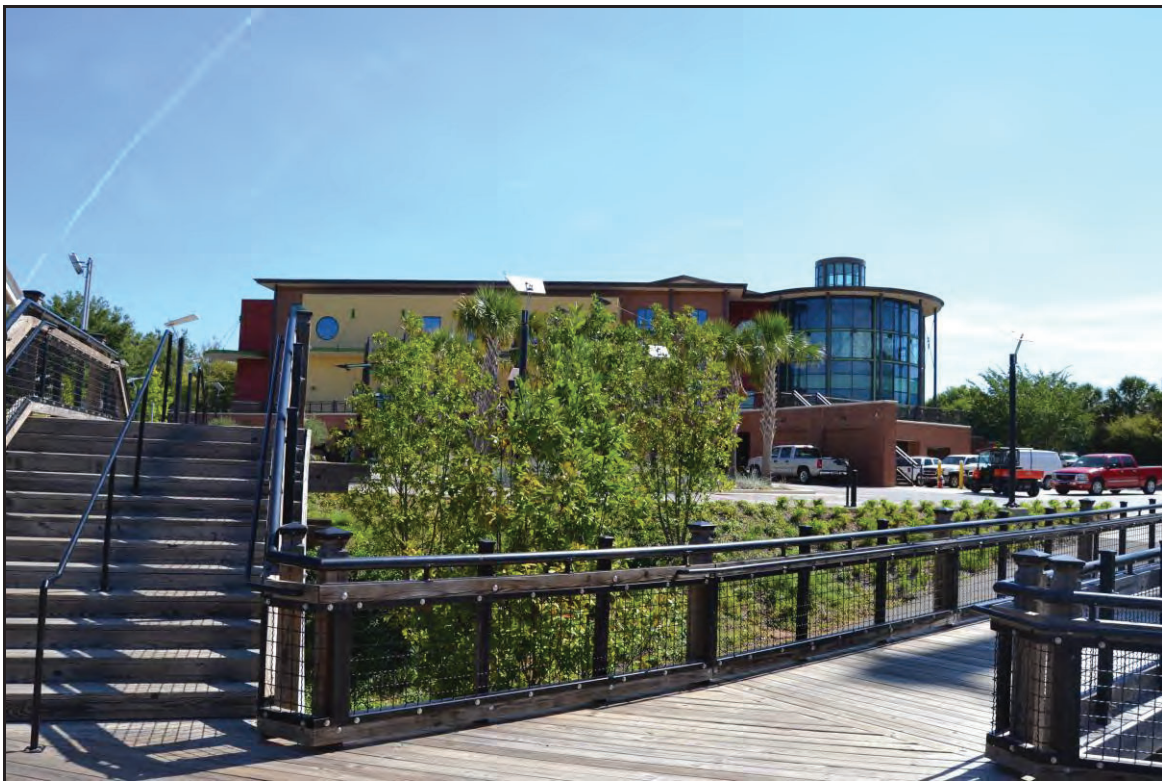
Figure 24. Example of modern buildings adjacent to the Canal Hydro Plant.
