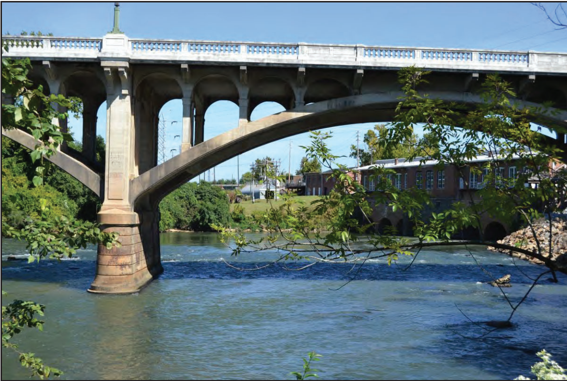
Figure 22. View from project location to Canal Hydro Plant, facing north.
